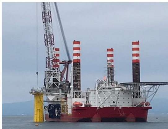
Projects in Akita Port and Noshiro Port (offshore)
