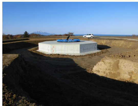
Hokkaido: Kamiyuchi Project (onshore)
