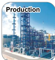
Production plant newly built on premises of Cosmo Oil's Sakai Refinery
