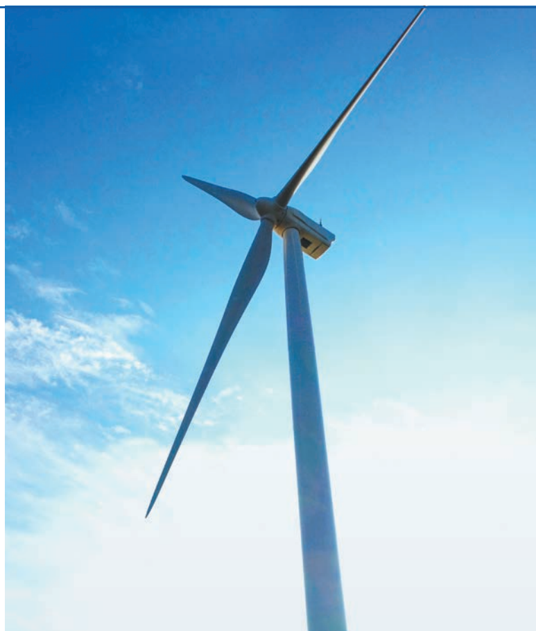
Wind power station (Sakata Port)
