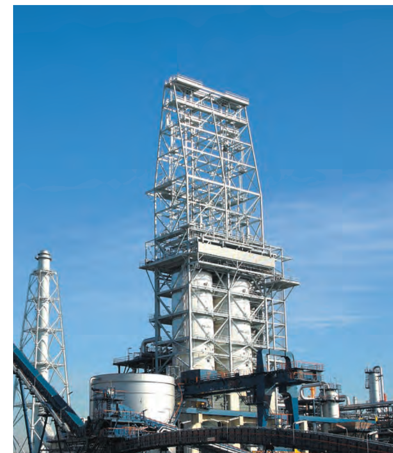
Delayed Coker (Sakai Refinery)
