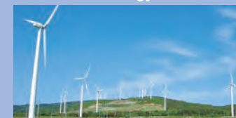
Wind power generation
