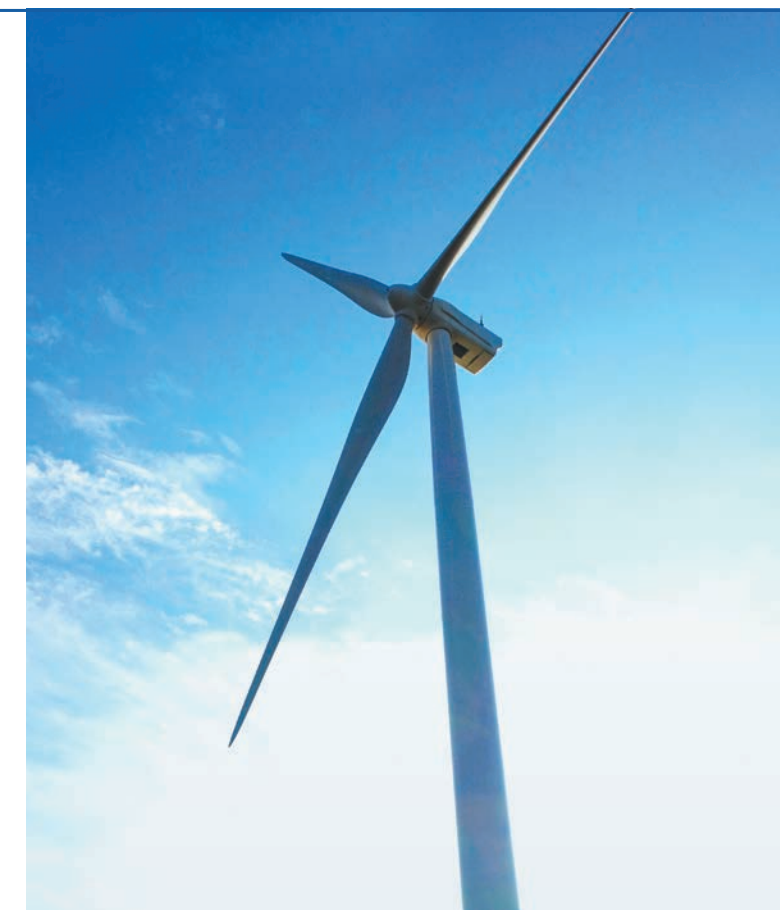
Wind power station (Sakata Port)
