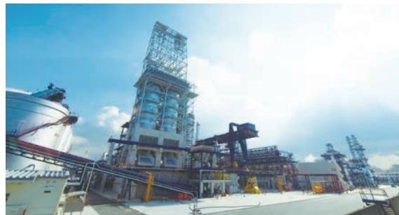
Delayed Coker unit at Sakai Refinery
