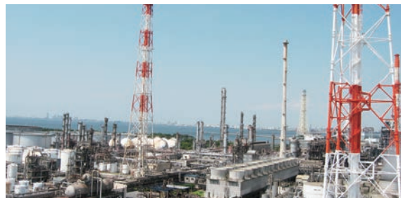
Maruzen Petrochemical's Chiba Plant
