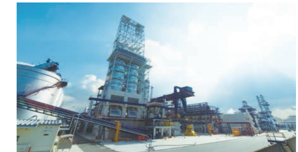
Delayed Coker unit at Sakai Refinery
