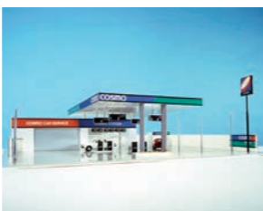
Cosmo Service Station redesigned
