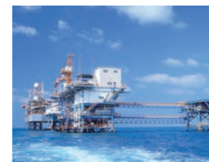
Offshore oil collection base for oil development
