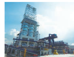
Delayed coker unit at Sakai Refinery
