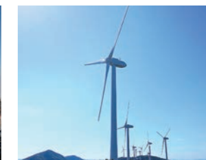
Wind power generation
