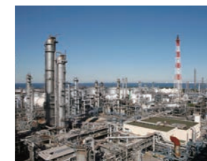
Maruzen Petrochemical's Chiba Plant
