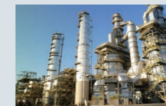
Para-xylene production facility
