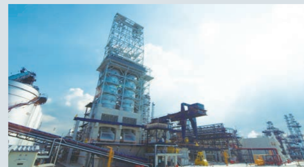
Sakai Refinery coker
