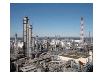
Maruzen Petrochemical's Chiba Plant
