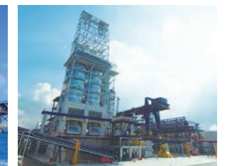
Delayed coker unit at Sakai Refinery
