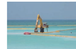
Installation of silt curtains
