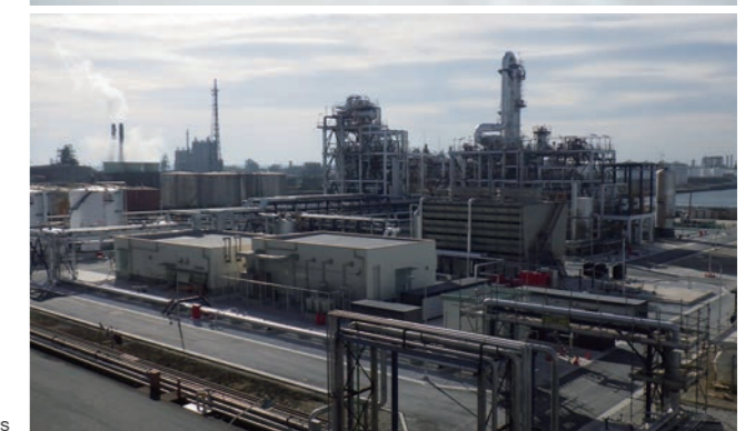
Production facility for hydrogenated petroleum resins
