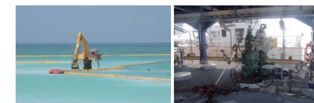
Installation of silt curtains
