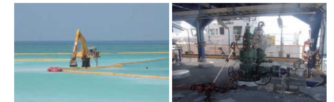
Installation of silt curtains
