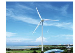
Wind power generation
