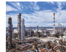
Maruzen Petrochemical's Chiba Plant
