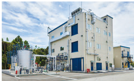
Cutting-edge photoresist polymer manufacturing facility exterior
