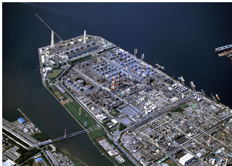
<Cosmo Oil Chiba Refinery>
