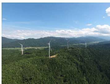
Tsurugamine Wind Power Plant
