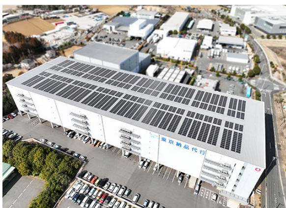
▪Exterior of Tokyo Nohin Daiko Narita FLC I
