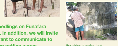
Repairing a water tank
