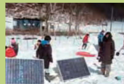
Students set up solar panels
