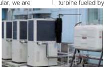
Kerosene heat-pump air-conditioning unit<sup>2</sup>
