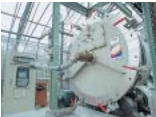
Experimental plant for slurry method biotechnological soil remediation
