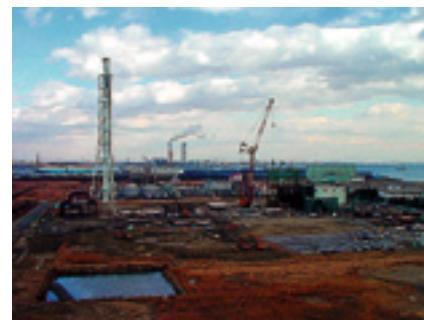
Power station under construction in Yokkaichi
