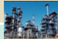
Diesel fuel desulfurization unit
