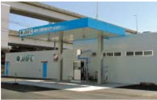
Hydrogen refueling station
