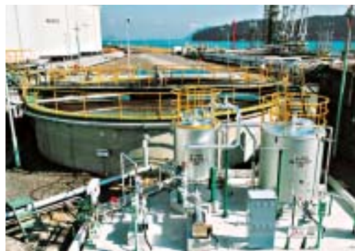
Wastewater treatment facility
