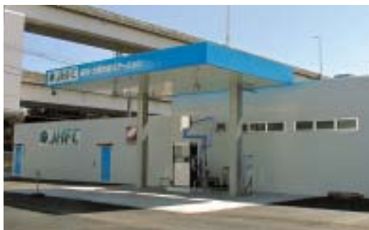
Hydrogen refueling station
