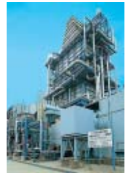
Co-generation unit at the Chiba Refinery
