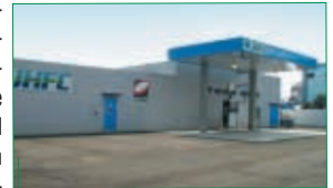
JHFC Yokohama Daikoku Hydrogen Station
