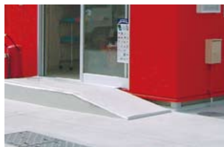
Wheelchair access ramp
