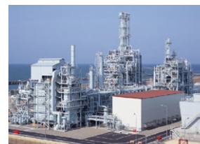
GTL demonstration plant
