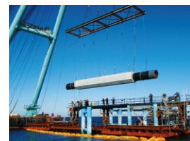
Restoration of ocean-bottom crude oil pipes
