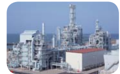
GTL demonstration plant
