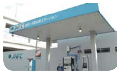
Yokohama-Daikoku Hydrogen Station
