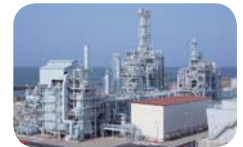
GTL demonstration plant
