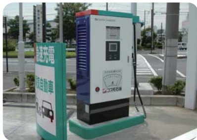
High-speed recharger for electric vehicles
