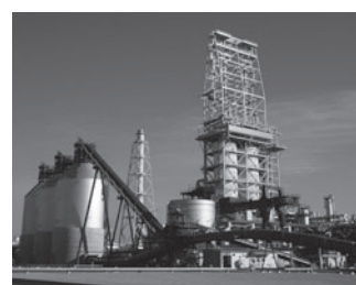
Delayed coker (heavy oil cracking facility)
