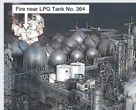
■ Figure 4. Ignition of leaking LPG and fire
