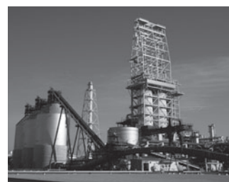
Delayed coker (heavy oil cracking facility)
