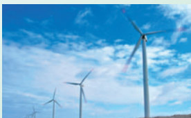
Hazaki Wind Farm
