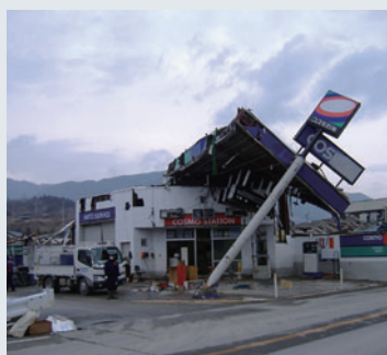
Service station damaged due to March 11 quake (taken on March 25, 2011)
