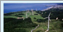
Reuke and Rumoi Wind Farms Total output capacity: 5,360 kW No. of turbines: 10
