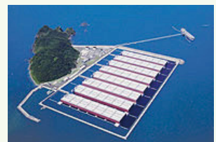
Oil storage site
