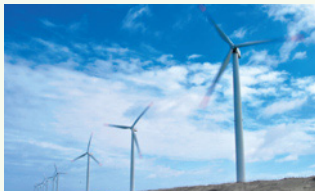
Hazaki Wind Farm
