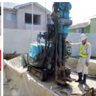
▲ Soil sampling by boring
