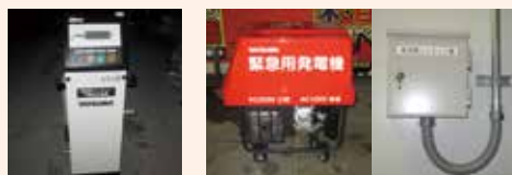
From left: Portable fuel pump, emergency power generator, connection box for emergency power generator
