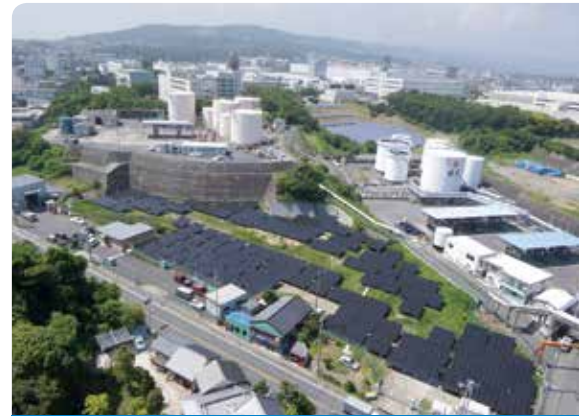
Hitachi Solar Power Plant (CSD Solar)
