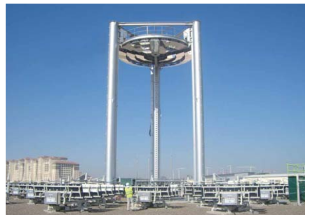
▲ Pilot plant in Masdar City for testing the "beam-down" type solar concentration system
